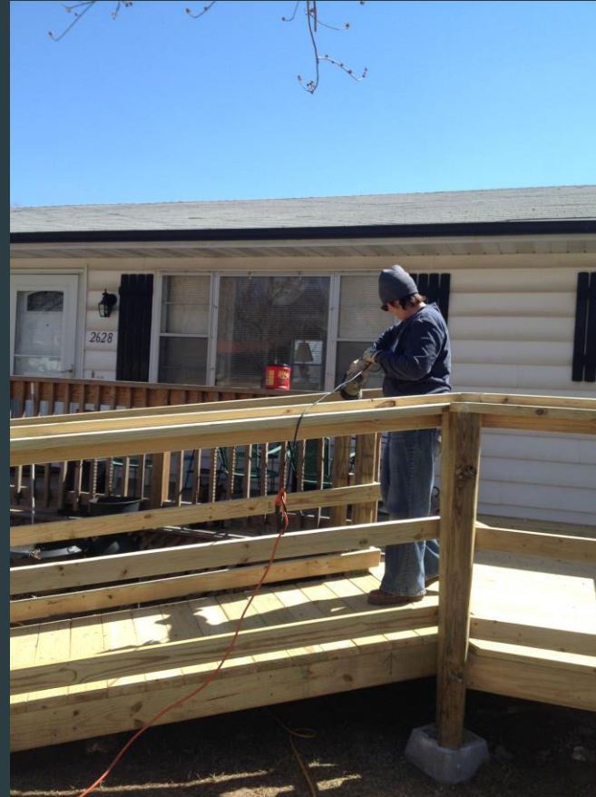
Sanding the Final Finish for the Ramp
