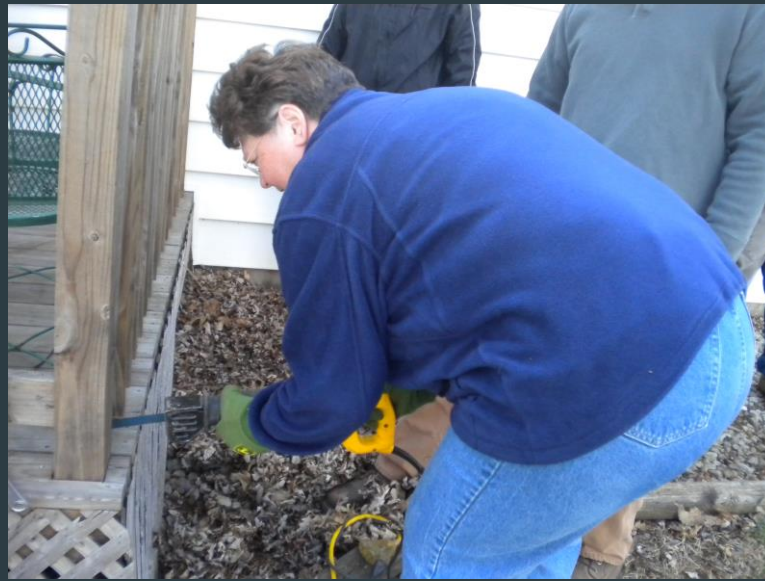
Charlyce taking a saw and sawing the posts
